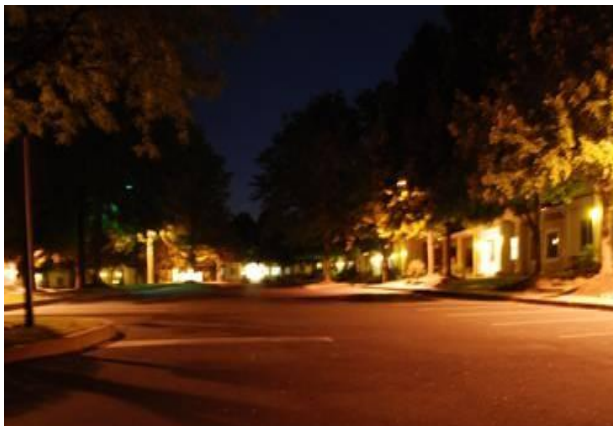
250w HPS (296 system watts)
