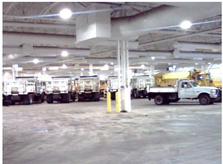
100w replacing 400w MH
